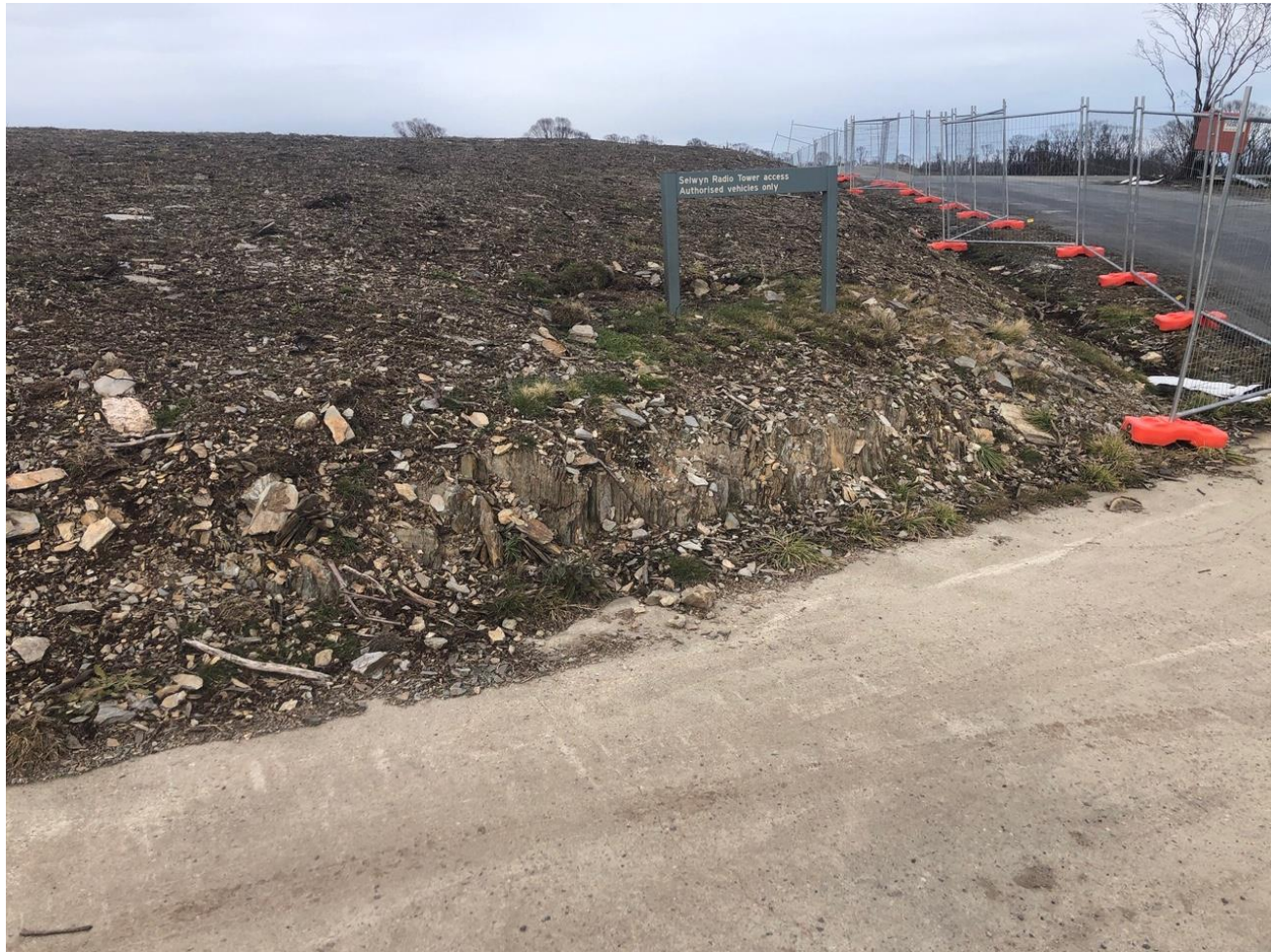
Photo 6 – 10/7/2020 – View of an existing cutting on the corner of Kings Cross Road and Selwyn Trail (near NW corner of the proposed Guest Facilities building), showing slate bedrock at shallow depth.
