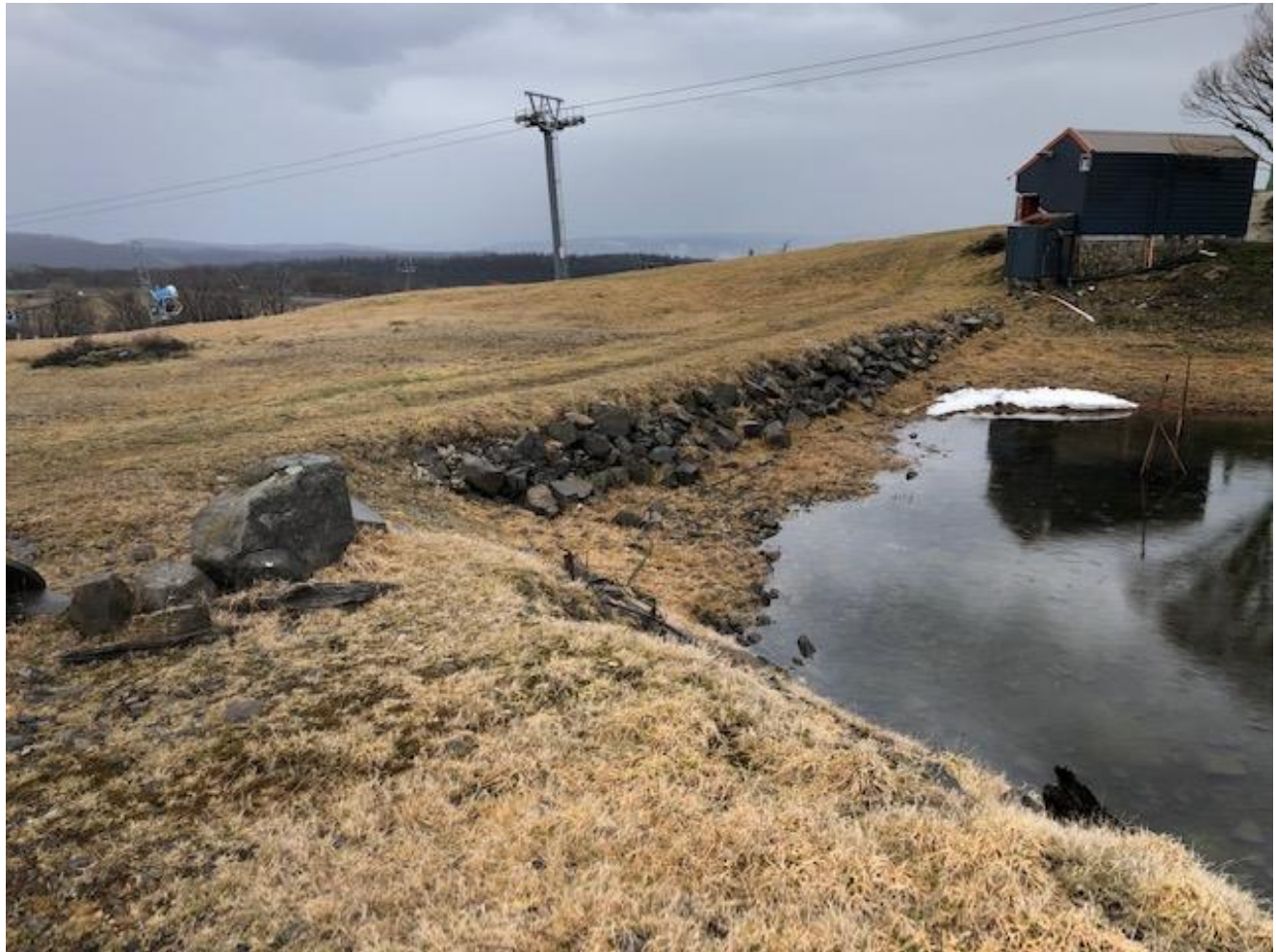
Photo 12 – 18/9/2020 – View of the quarry that is being used as a water storage dam. A retaining wall will be constructed along the downstream end to increase the water holding capacity.
