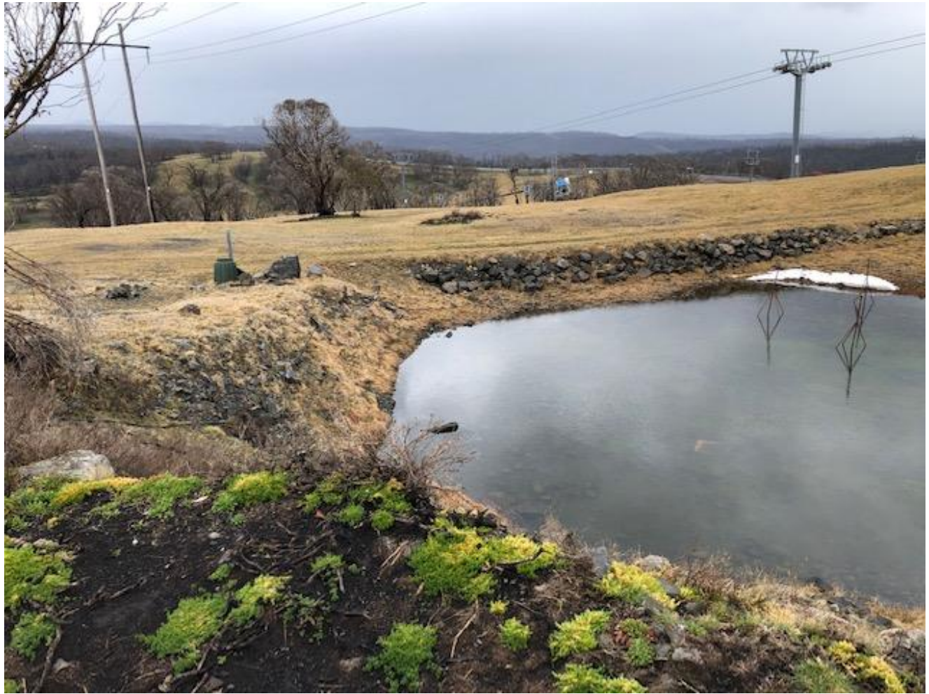
Photo 13 – 18/9/2020 – View of the quarry that is being used as a water storage dam. A retaining wall will be constructed along the downstream end to increase the water holding capacity.
